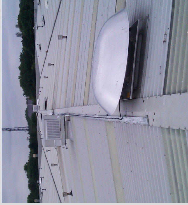
Tornado can be combined with the Colt CoolStream evaporative cooler to provide cost-effective air conditioning for industrial and commercial applications
