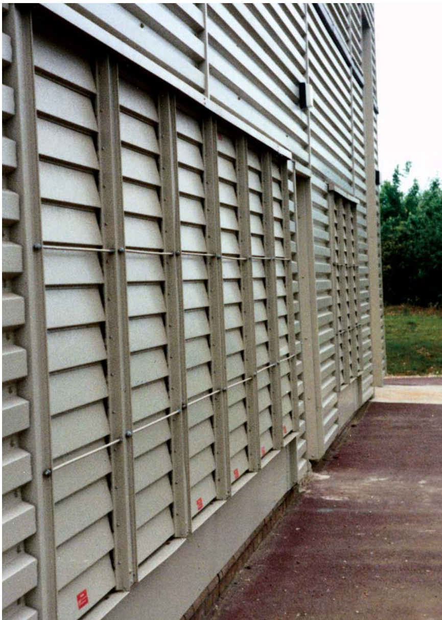
Above - Seefire natural ventilators installed into a near vertical position.
