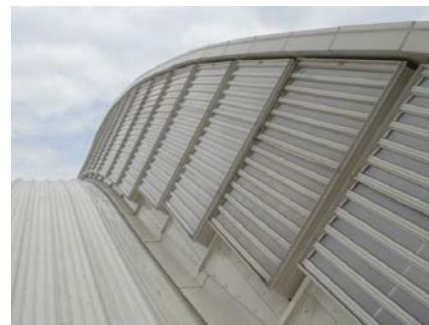
Above - Seefire natural ventilators installed into a near vertical position.
