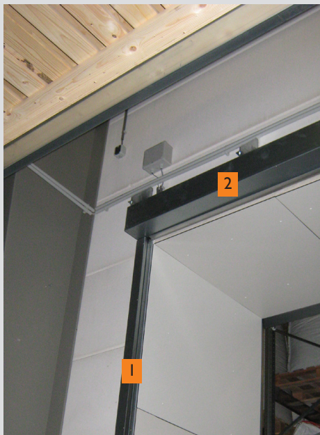
Side guides (1) and headbox (2). All unit components have been completely polyester powder coated
