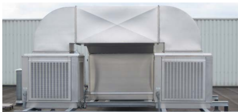
Typical ductwork layout showing two CoolStreams in tandem with re-circulation of air through a Coltair de-centralised air handling unit.
