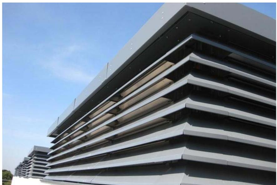
*Roof top double bank louvre turrets with internal controllable dampers to regulate the flow of air and eliminate rain entry.*
