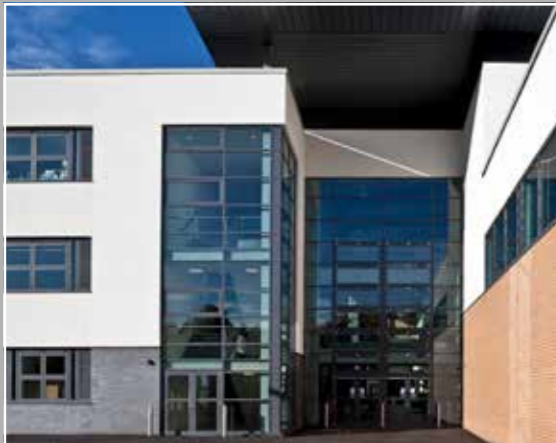
Auchmuty High School in Fife now benefits from our day-to-day ventilation and smoke extraction systems.
