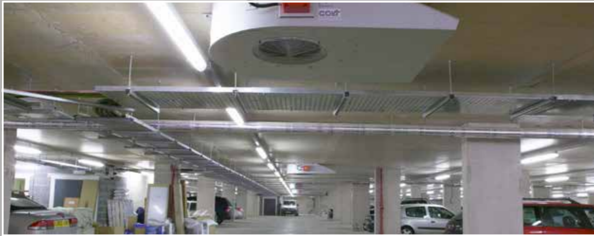
Colt Cyclone's low profile design and high velocity induction fan reduces the concentration of polluted air in car parks.
