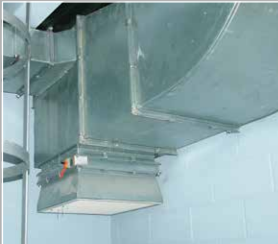
Our pressurisation systems are designed to keep fire-fighting shafts and staircases clear of smoke.
