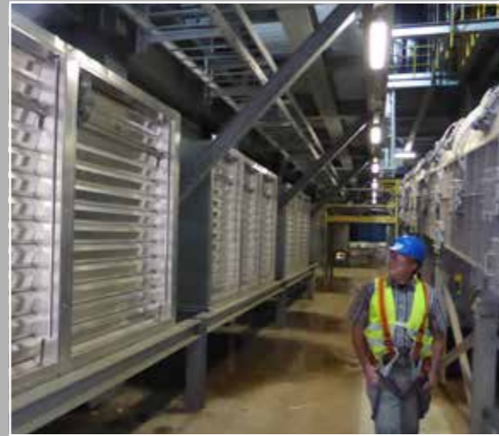
As the pioneers of smoke control, Colt's design support is second to none.
