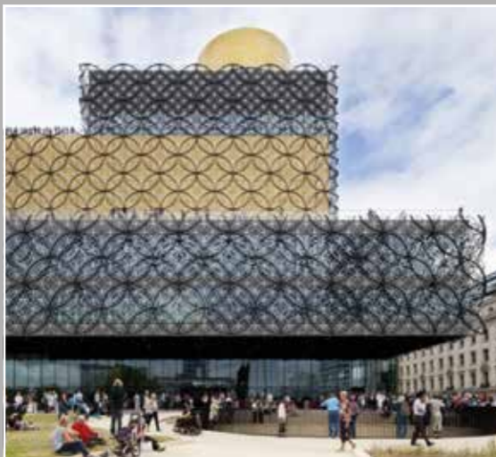
Colt provided smoke control for the Library of Birmingham, incorporating Coltlite and CoolShaft systems.
