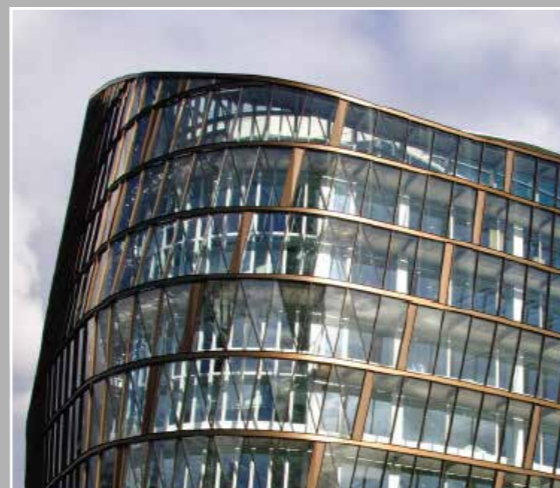
We supplied the Co-operative Group headquarters in Manchester with day-to-day and smoke ventilation.
